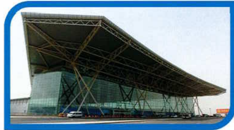
Tianjin Binhai International Airport
