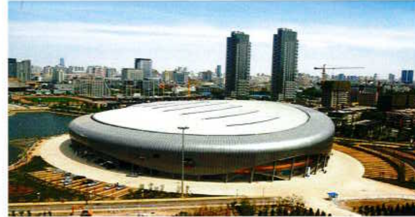
Tianjin Olympic Center (Aquatics)
