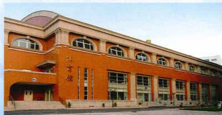
Tianjin Foreign Studies University Gymnasium (Fencing)
