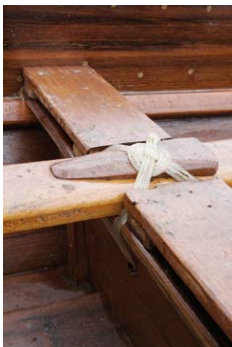
Picture 6: Tightened ropes connect the spine to seats and bulkheads
